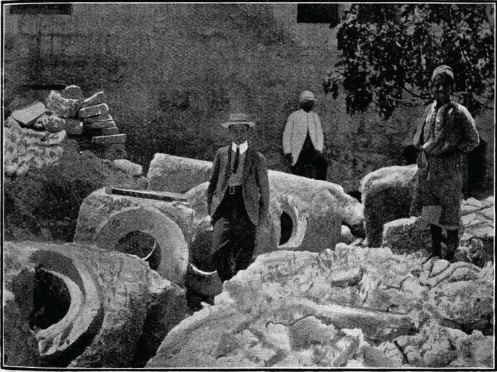
FIG. 1.—Disjunct Tubes of the Stone Syphon.
