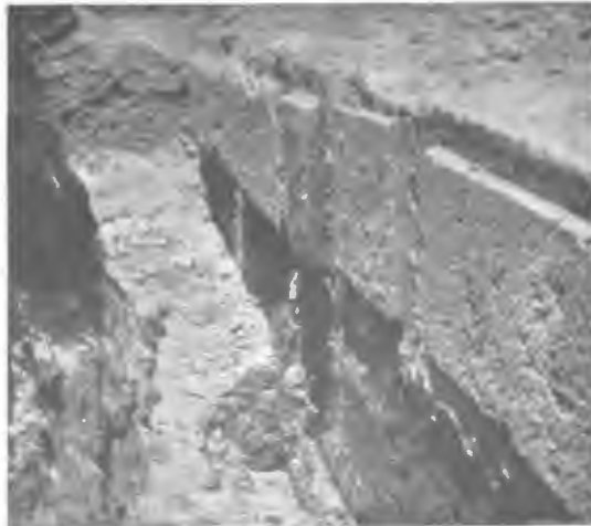
11. WESTERN PIER: WEST FACE.
