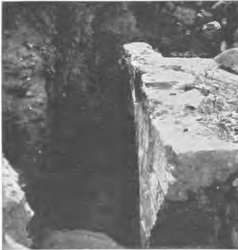
9. WESTERN PIER, FROM THE NORTHEAST.
