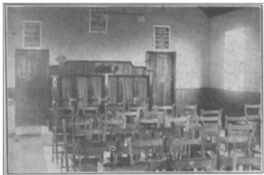
ELIM HALL HADLEIGH (INTERIOR)
