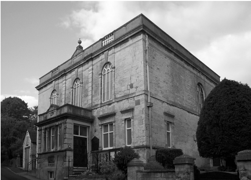
Christ Church (Baptist/URC), Painswick, Gloucestershire, built in 1803 it was renamed the Cornelius Winter Memorial Chapel in 1892.
