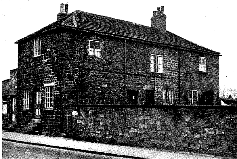
THE FIRST THORNER CHAPEL, BUILT c. 1762. (Now two cottages.)
