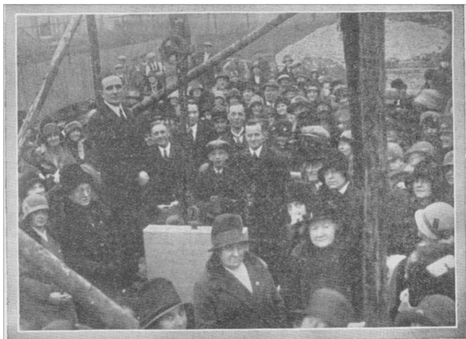
Principal George Jeffreys laying the Foundation Stone of the new Elm Tabernacle at Lastbourne in 1929. This Tabernacle is now a flourishing centre of Foursquare revival.
