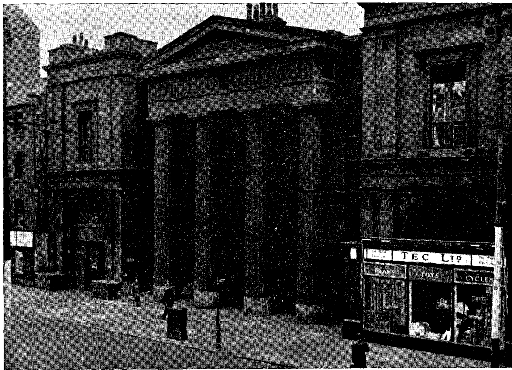
THE FORMER BRIDGE STREET CHAPEL, GLASGOW, showing the handsome portico, recently demolished.
