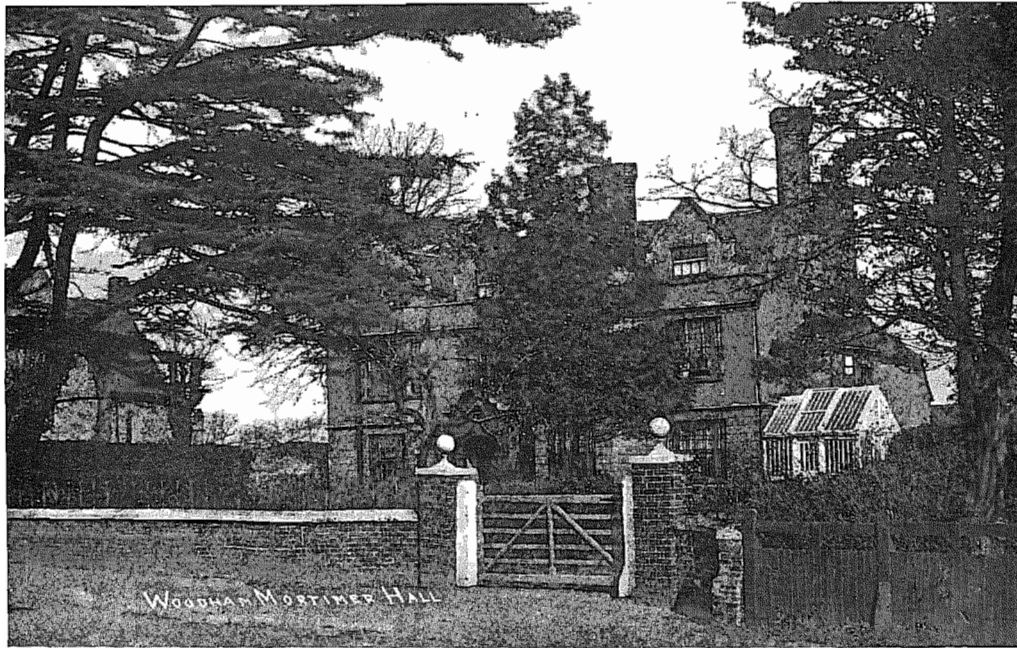
WOODHAM MORTIMER HALL, MALDON, ESSEX, where Dr. Peter Chamberlen (1601-1683) passed the later years of his life. Behind the cedar tree, on the left side of the picture, one may see the East end of the church. In the North-east corner of the churchyard, quite near to the Hall property, stands the monument which marks the Doctor's last resting-place—"the grave my hardest, but my easiest bed."
