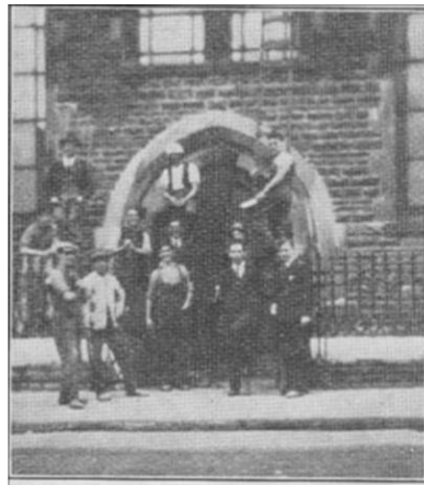
Renovating Elim Tabernacle, Swansea
