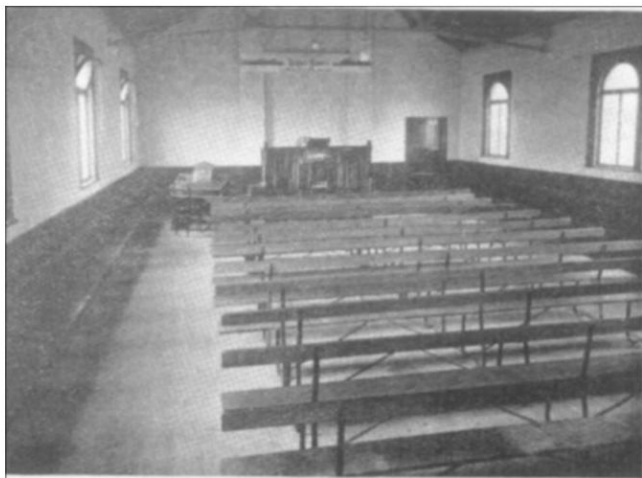
INTERIOR OF THE NEW ELIM HALL, ESBARN
