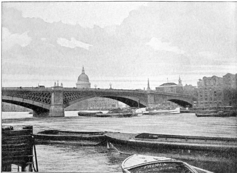
Figure 7. Southwark Bridge (Courtesy of Institution of Civil Engineers)
