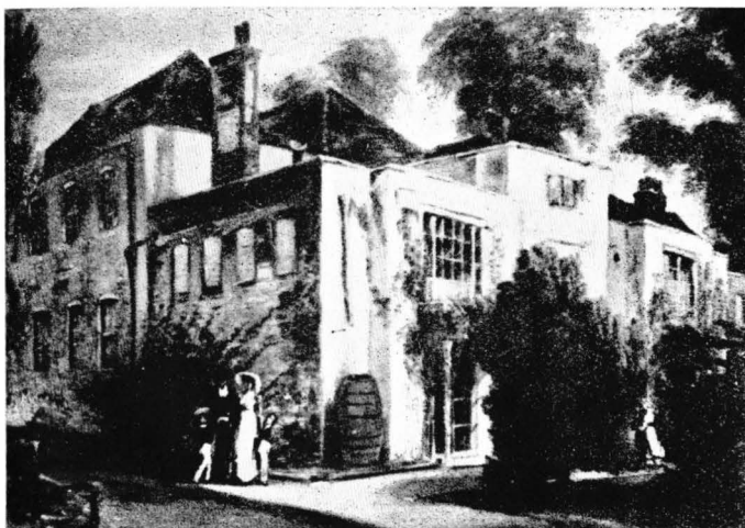
RIDGWAY HOUSE (original habitation of Mill Hill School).
